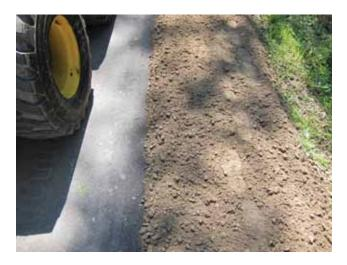
Figure 61: Ensuring Material is Above Road Surface
