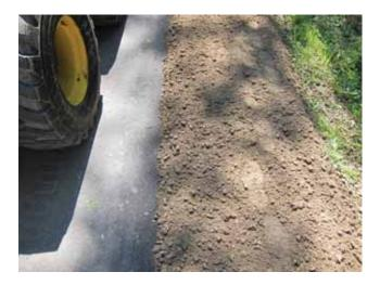
Figure 45: Ensuring Material is Above Road Surface
