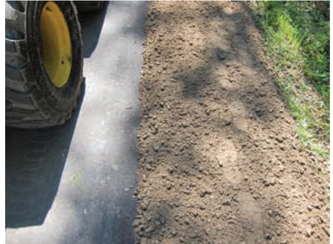
Figure 63: Ensuring Material is Above Road Surface
